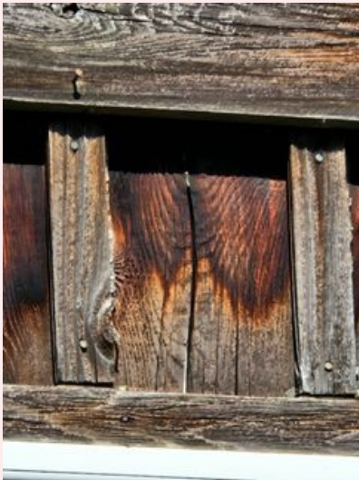
The south siding is splitting and could allow water entry
