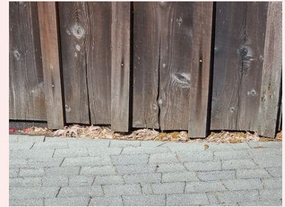
Water can get trapped between the trim and the siding. There is a risk of concealed decay and some of these details.
