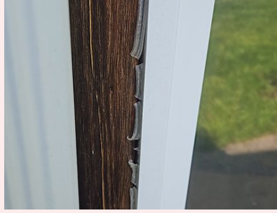
Failing a sealant noted between Windows and trim at the east side
