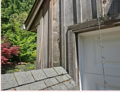
Damaged siding noted at the West face of the garage
