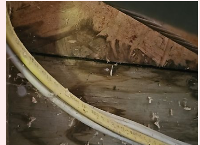
Water stains on the OSB sheathing beneath the electric panel are an indication that the siding could be leaking onto the sheathing in places.
