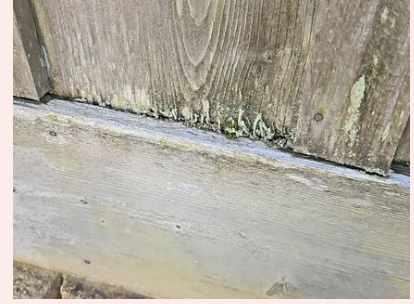
Water can get trapped between the trim and the siding. There is a risk of concealed decay and some of these details.
