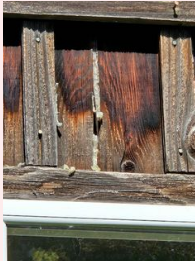
Sealant failure noted everywhere
